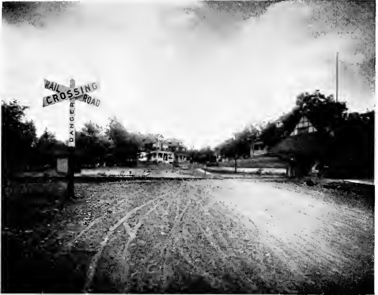
DANGEROUS GRADE CROSSING AT ERIE STATION
